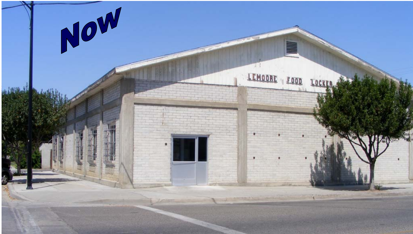
Lemoore Food Locker New Paint, Awning, Fascia and Signage
